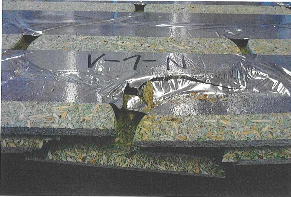
Fig. 6: Local punching failure (view after removing of cement-bonded board).
